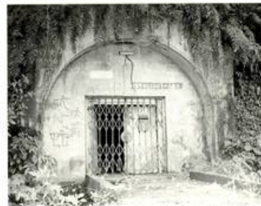
The Tunnel used for Taiwanese aborigine "Comfort Women"
